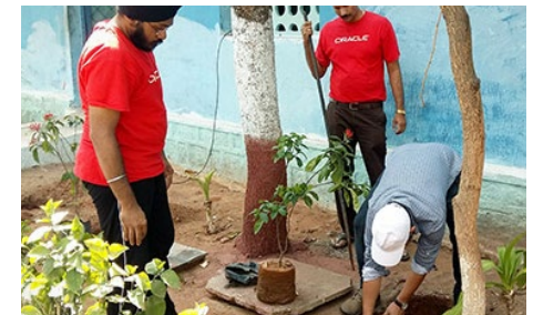
Building a Rainwater Harvesting Pit: Hyderabad, India
